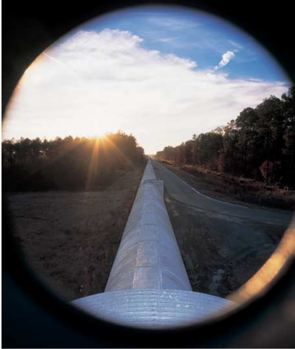
STRAIGHTER THAN THE SURFACE OF THE EARTH , the concrete tunnel that houses the west arm of the LIGO Livingston Observatory rises several meters off the ground on its four-kilometer run as the planet curves beneath it. The tunnel houses an airtight steel pipe. Inside the pipe is a vacuum, and through the vacuum shines a beam of infrared light with the power of 20 million laser pointers.
